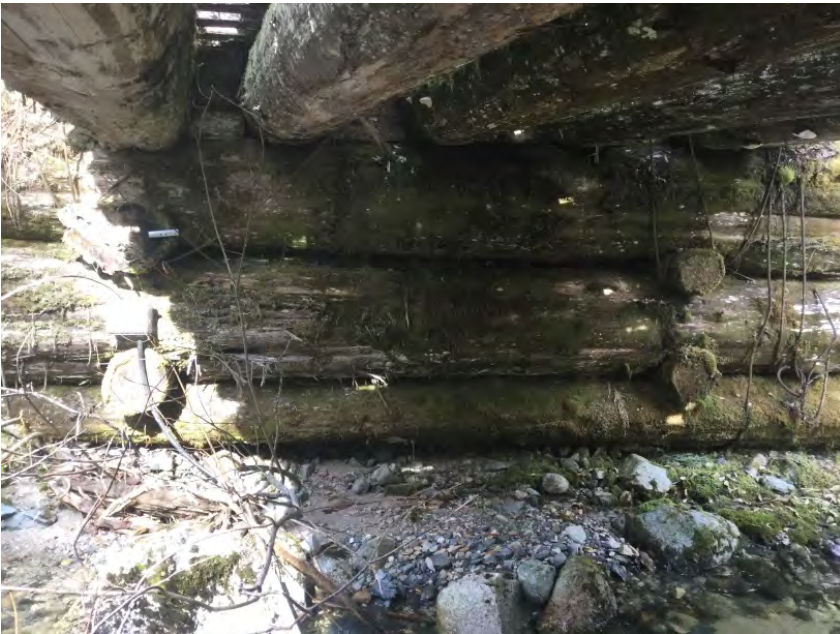
Left Bank Abutment when facing downstream
