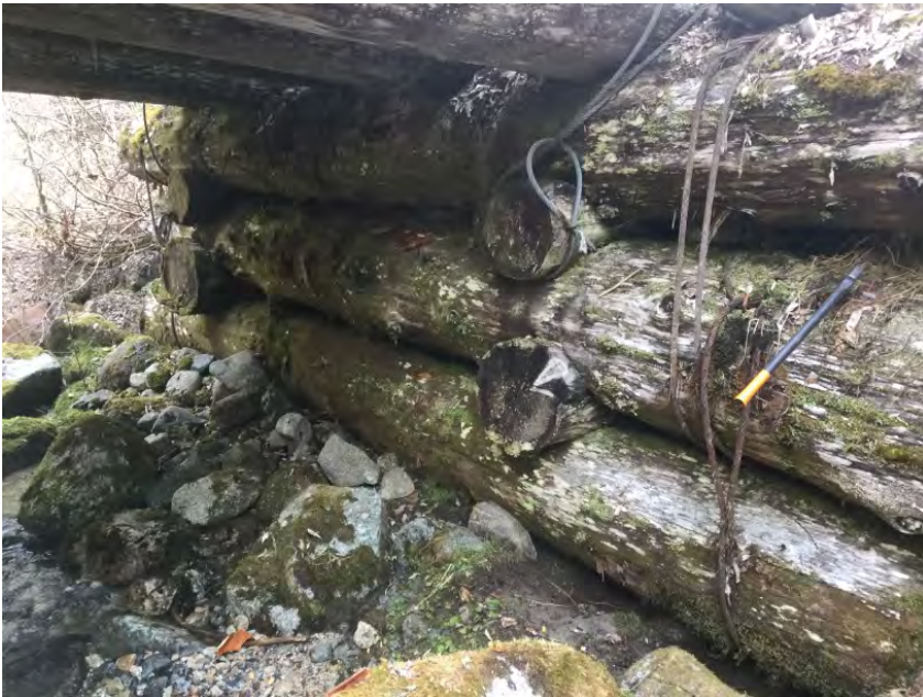
Right Bank Abutment when facing downstream
