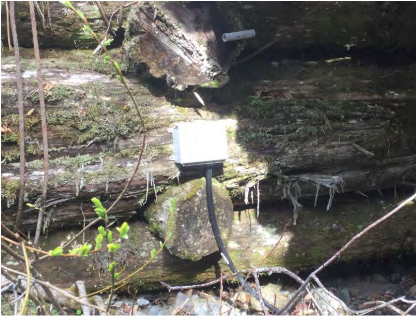
Water gauge under bridge and attached to left abutment
